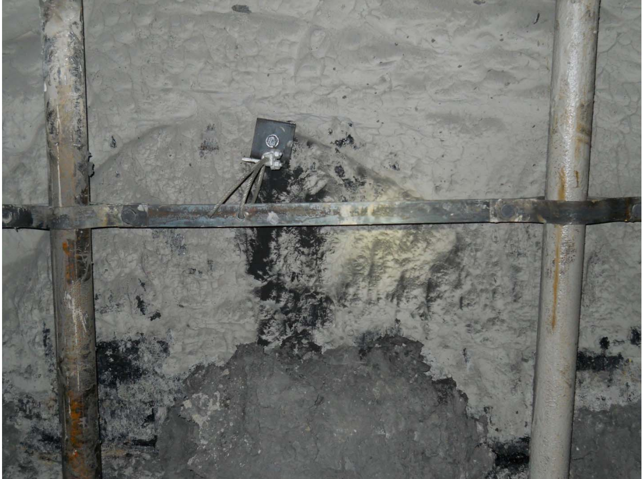
Photo of Supports that were Secured after the Accident
