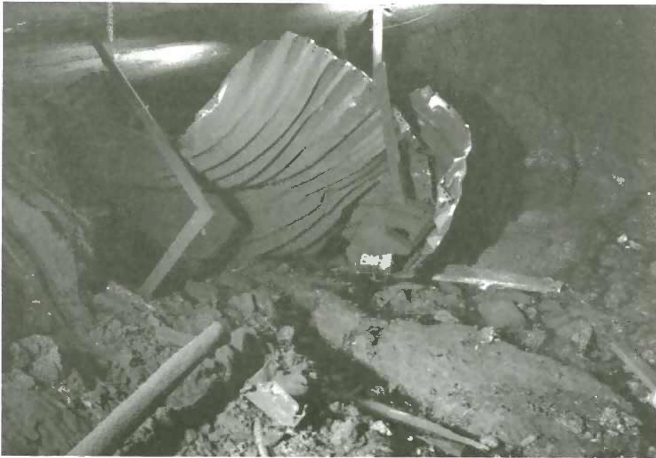
FIGURE 11. - Overcast destruction No. 64 x cut No. 7 slope.
