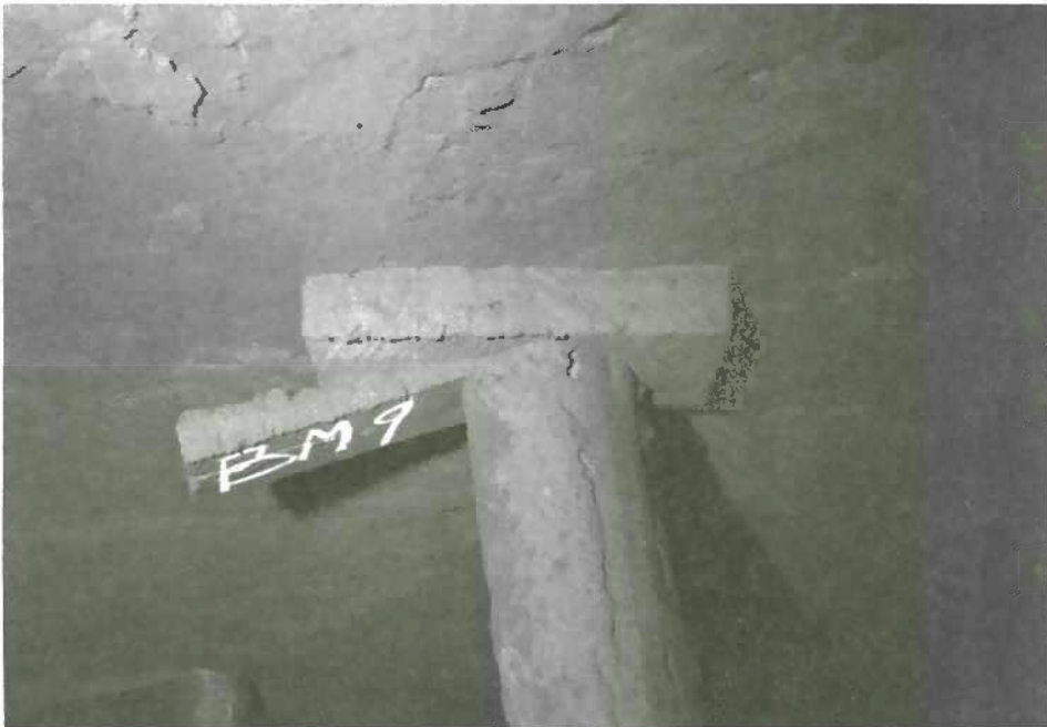
FIGURE 12. - Heavy coke on post about 20 ft outby last open x cut No. 2 entry 102 section.
