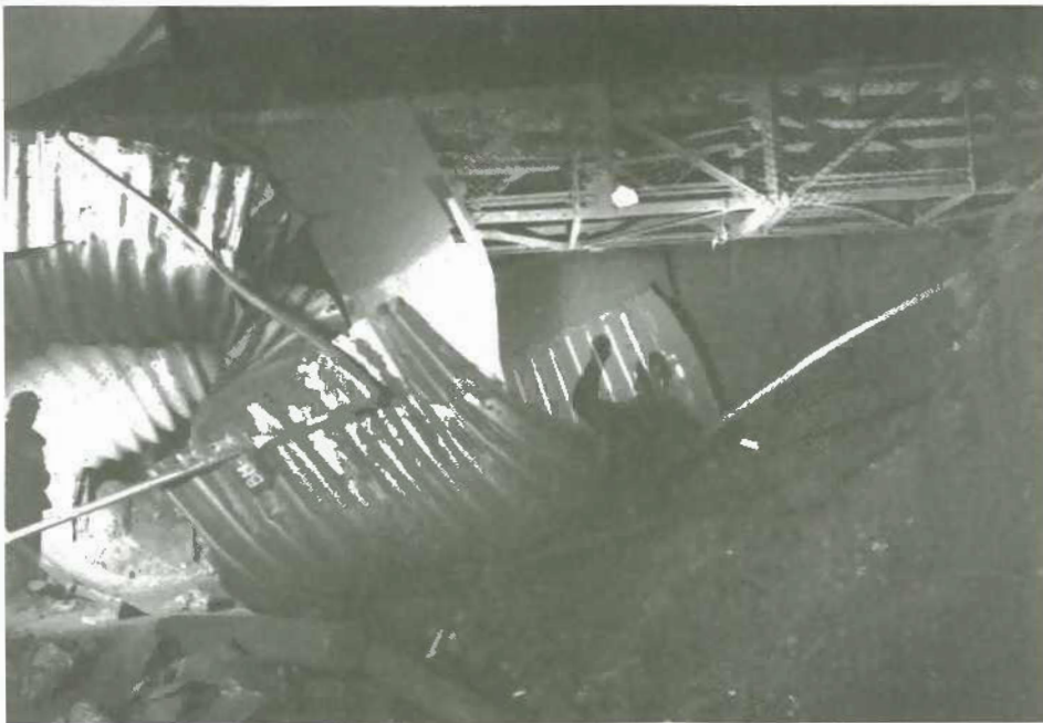
FIGURE 10. - Overcast destruction No. 5 slope No. 63 x cut.
