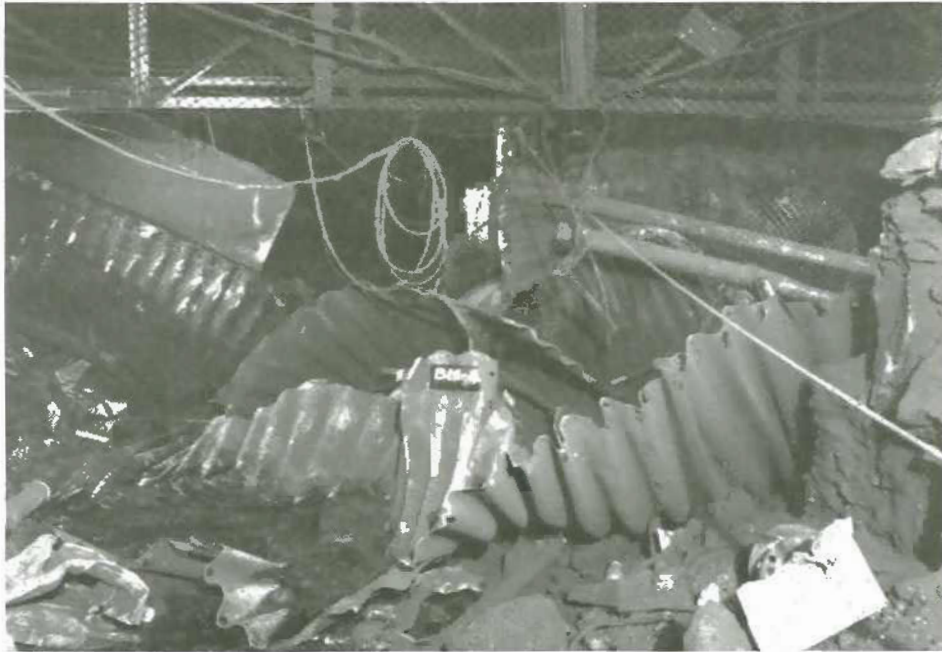
FIGURE 9. - Overcast destruction No. 6 slope 63 x cut.
