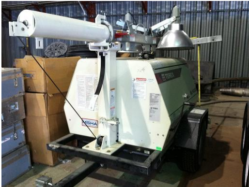
Tower and Generator for Repeater
