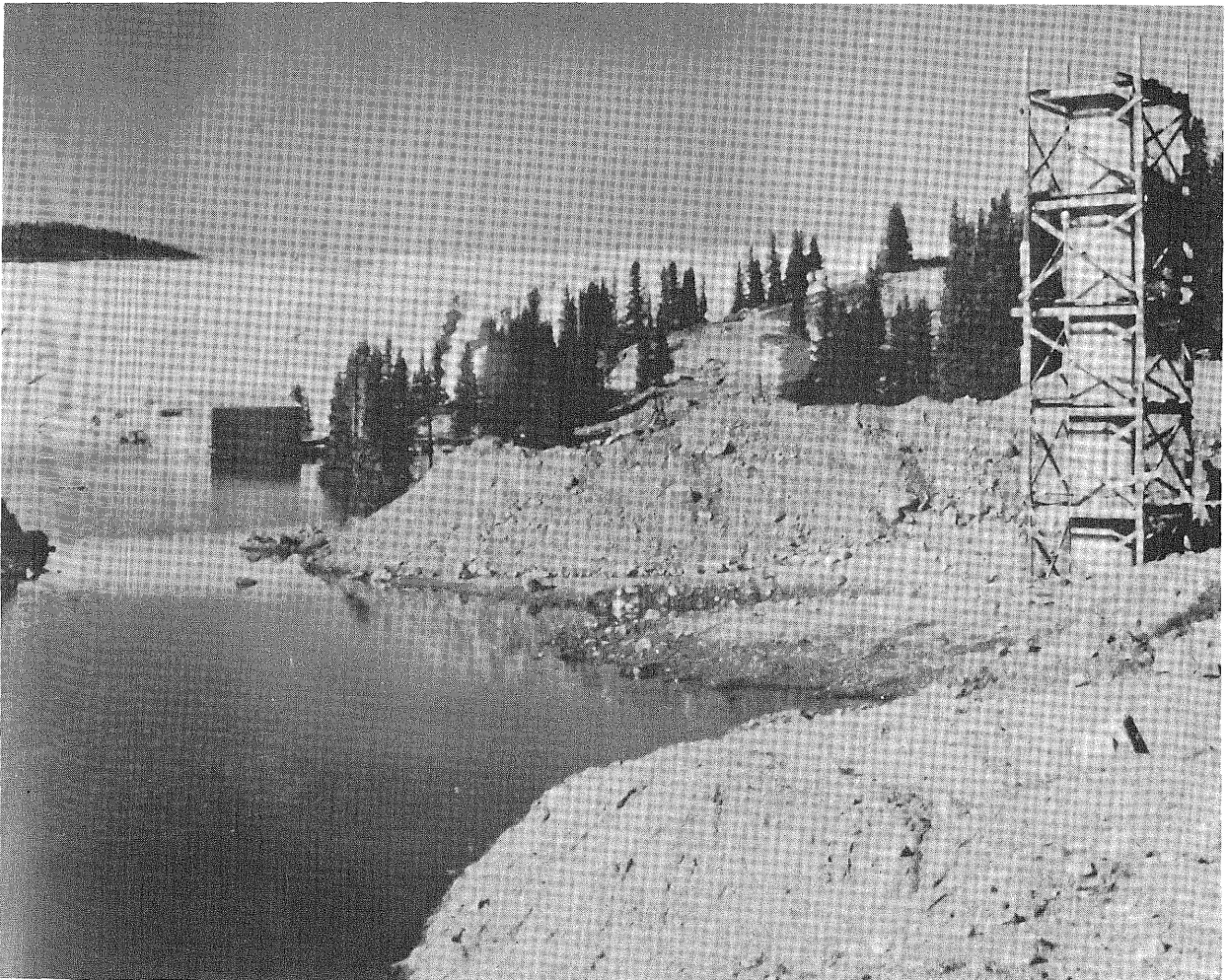
FIGURE 21. - Barge pump and decant tower in the same pond.
