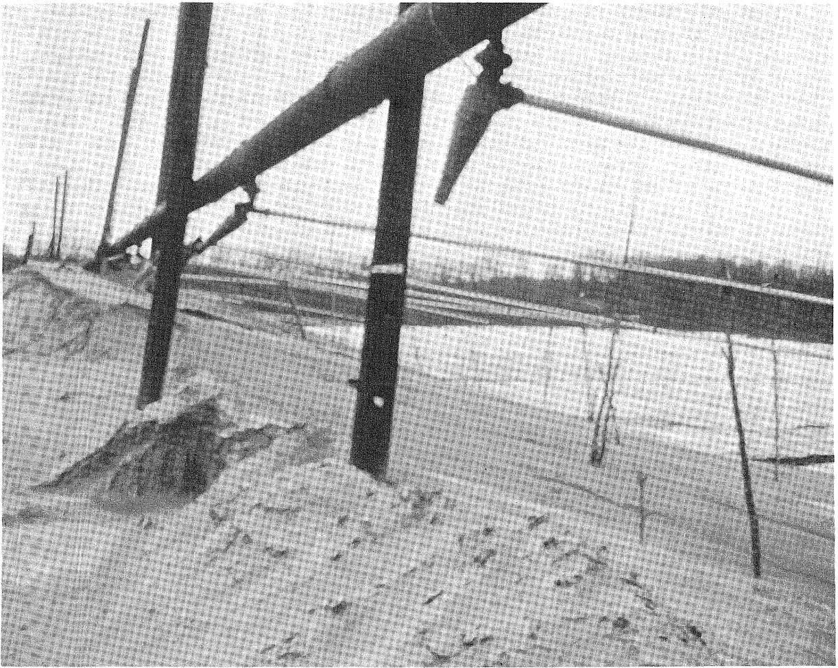
FIGURE 33. - Cyclones on centerline method of dam building in small operation.
