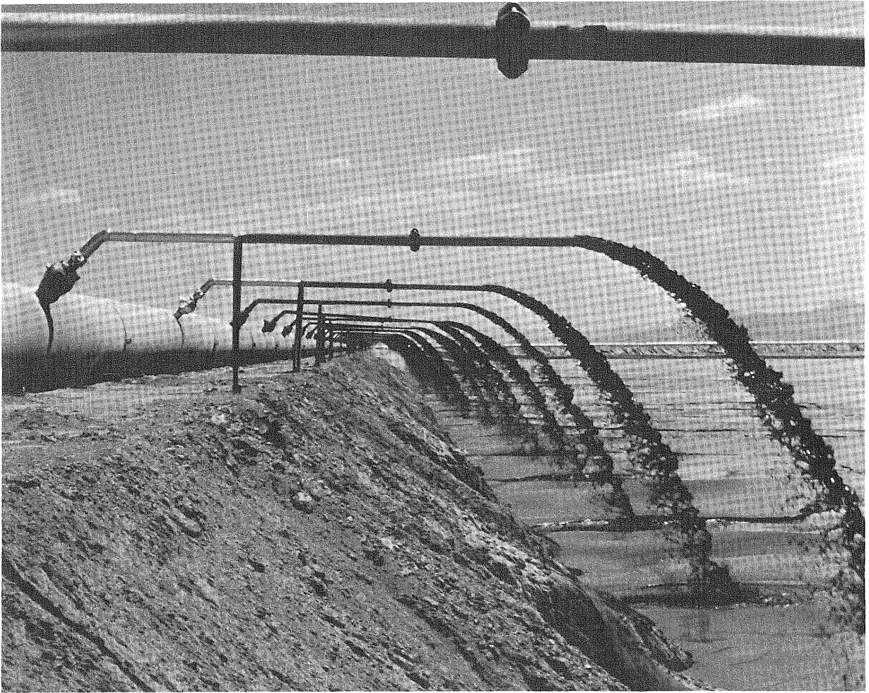
FIGURE 28. - Spigoting around periphery of dike—upstream method.
