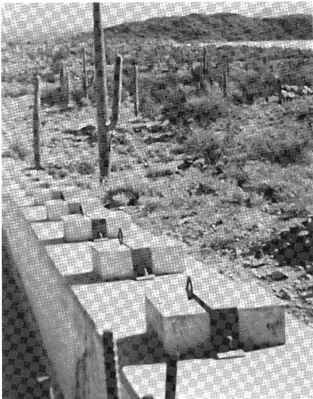
FIGURE 18. - Decant line to tower 6-inch outlets at each 6-inch elevation rise.
