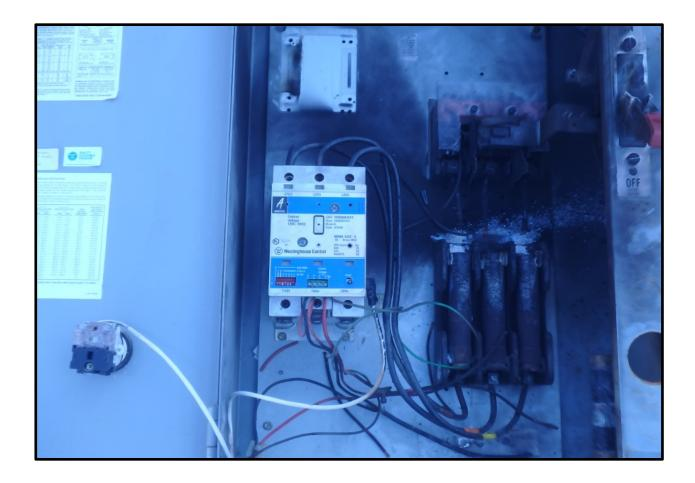
An electrician was working on an energized three-phase electrical circuit for a water pump. After replacing a blown fuse, the electrician noticed the pump motor was single-phasing. While attempting to attach the third phase, he accidently dropped the wire across an energized lug. The electrician received a severe flash burn to his hands..
