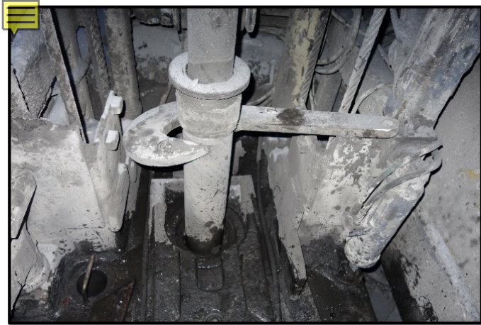
The drill motor turned unexpectedly, pinning the driller's leg between the tool and the drill mast.
