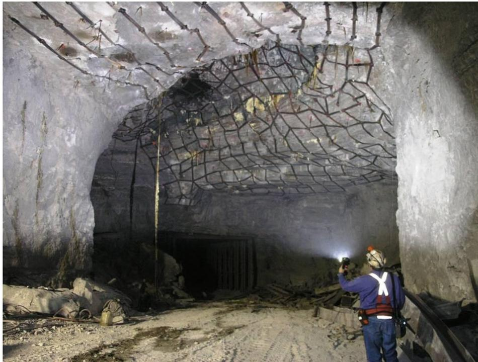
**Figure 28.** Bolts, straps, and injection grouting used to rehabilitate the roof at the site of a major roof fall.
