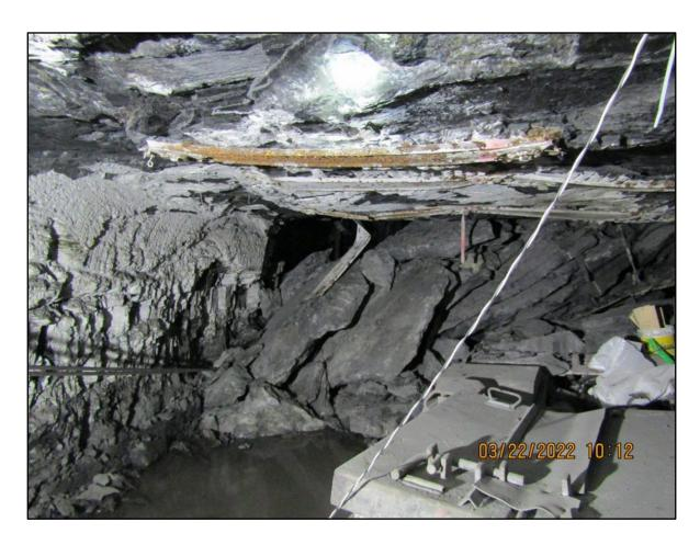
A miner died when he was struck by a roof fall outby the retreat mining section. The roof fall was approximately 40 feet long, 18 feet wide, and five feet thick.
