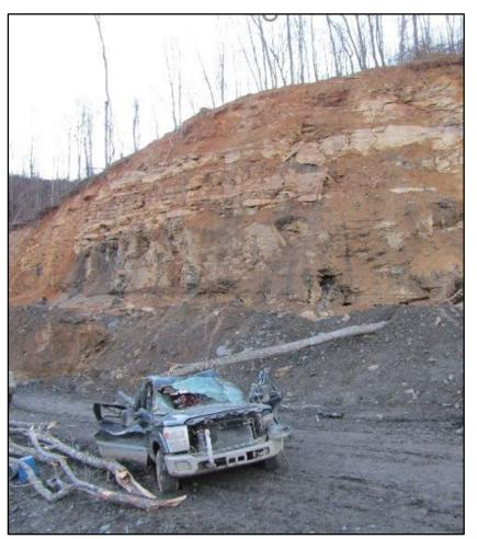
A blaster died when a tree fell from the highwall adjacent to the mine road and struck the cab of the pickup truck that he was driving.
