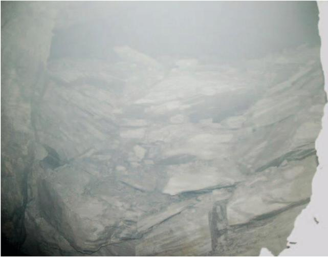
**Figure 5.** Roof fall debris is composed of very large blocks. The photo vantage point is approximately 40 ft from the rubble.
