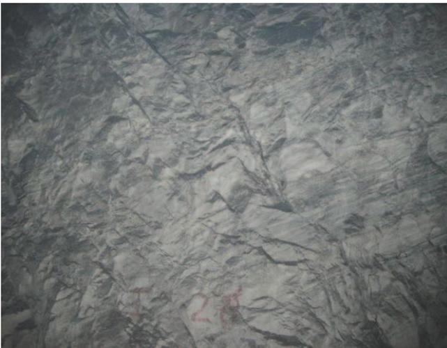
**Figure 6.** Open-aperture joint, which strikes N 10° W and dips 63° W, is located in the center of pillar II28. This orientation of joints typically runs diagonally from corner to corner in the JJ, II, and HH pillars. White outline represents close-up shown in Figure 7.
