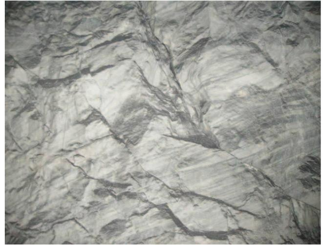
**Figure 7.** Close-up of Figure 6, showing open aperture along joint that penetrates deeply into the pillar. This feature contrasts with the irregular, localized nature of small fractures that represent blast damage on the pillar skin.
