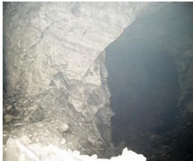
**Figure 4. The row of pillars at the margin of the benched area is characterized by extreme degradation, with the eastern portions (facing the benched side) 50 ft tall and exhibiting failure along pre-existing geological structures.**
