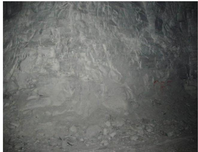
**Figure 8.** Typical condition of pillars on the 820-ft and 890-ft levels, showing an absence of open-aperture joints or evidence of raveling.
