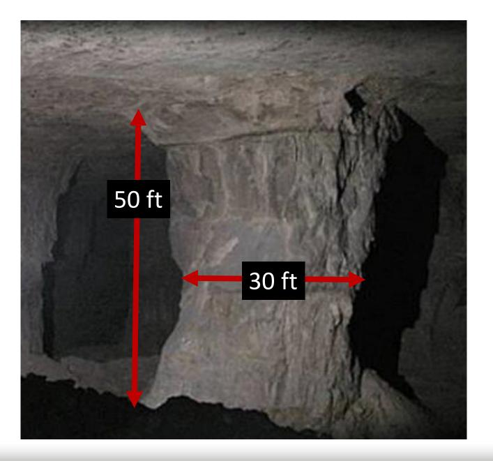
Slender Pillars, with width-to-height ratios less than 0.8, are at risk of collapse.
