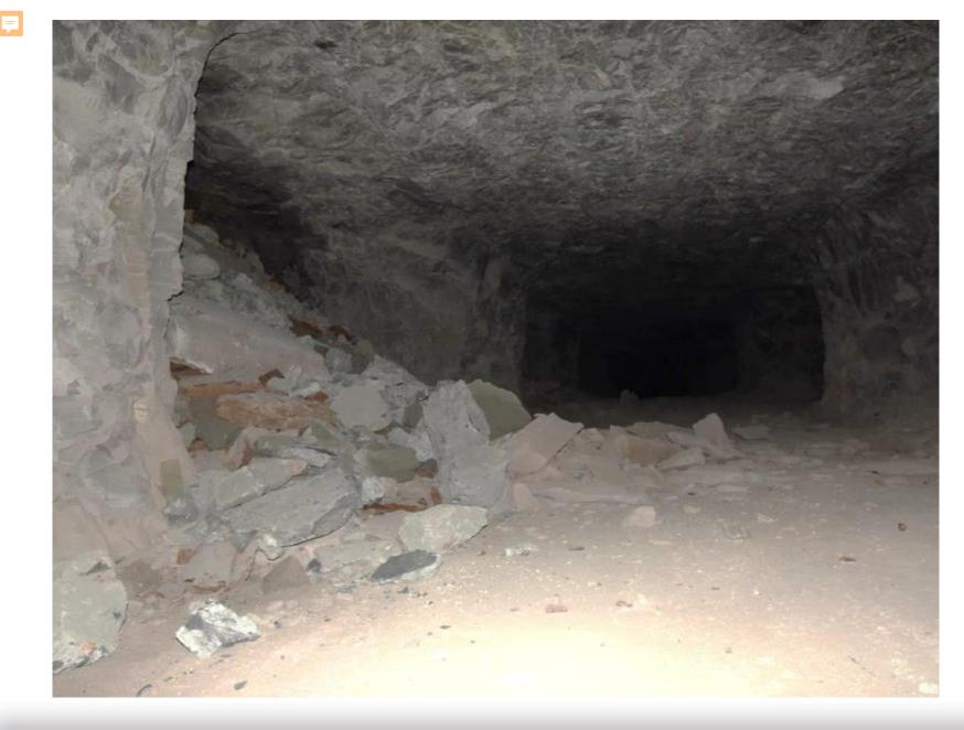
Miners working nearby a collapse, or traveling in an adjacent haulroad, could be killed or injured by falling rock or extremely high air velocities.
