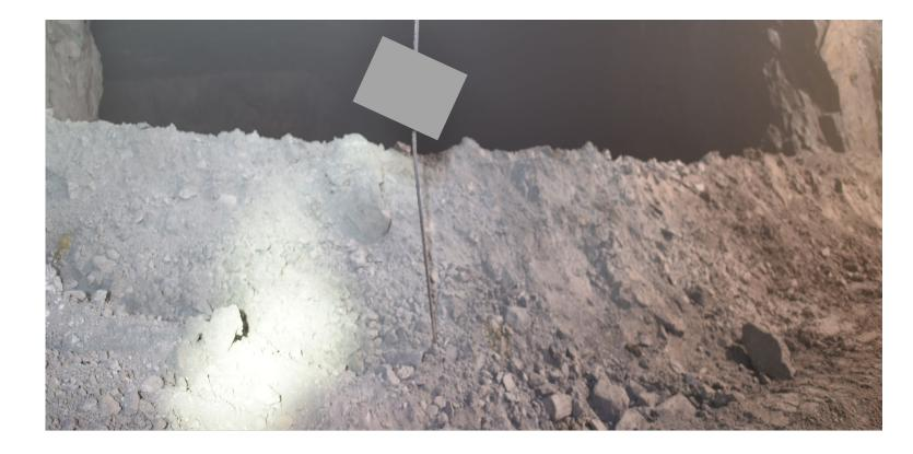
2. Construct bulkheads or rock barriers to redirect airblast away from miners.
