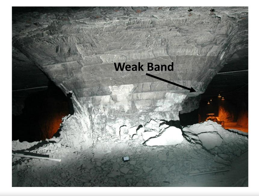
Weak bands or soft floor can cause rib slabbing and reduce pillar strength.
