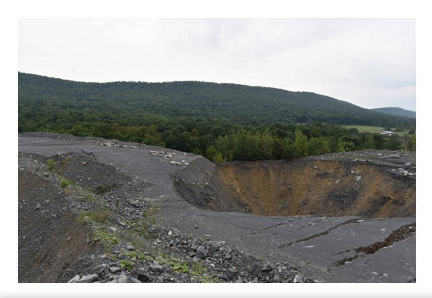
The total collapse of the overburden typically causes a subsidence feature (sinkhole) on the surface.
