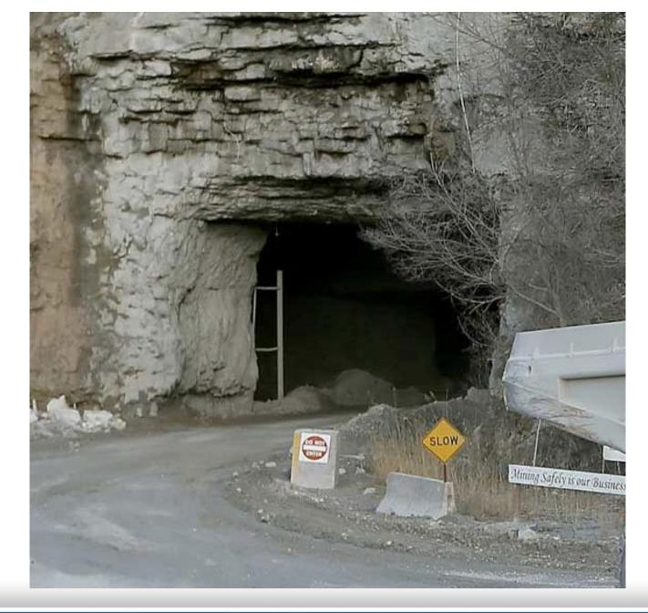
Airblast relief openings can provide a direct ventilation pathway that does not expose miners to the hazard.
